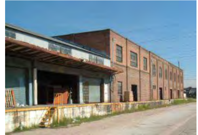
NFB Rentals Warehouse
