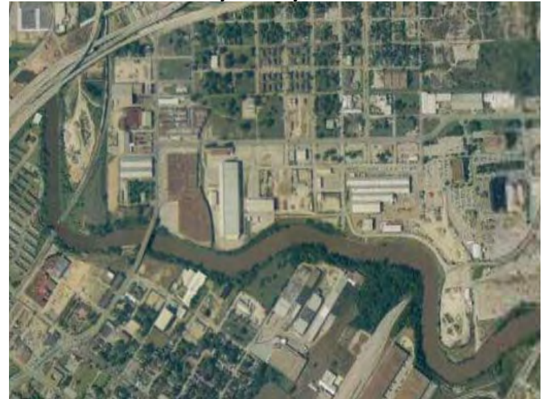
Aerial View of Zone 2 in the Buffalo Bayou Study Area
