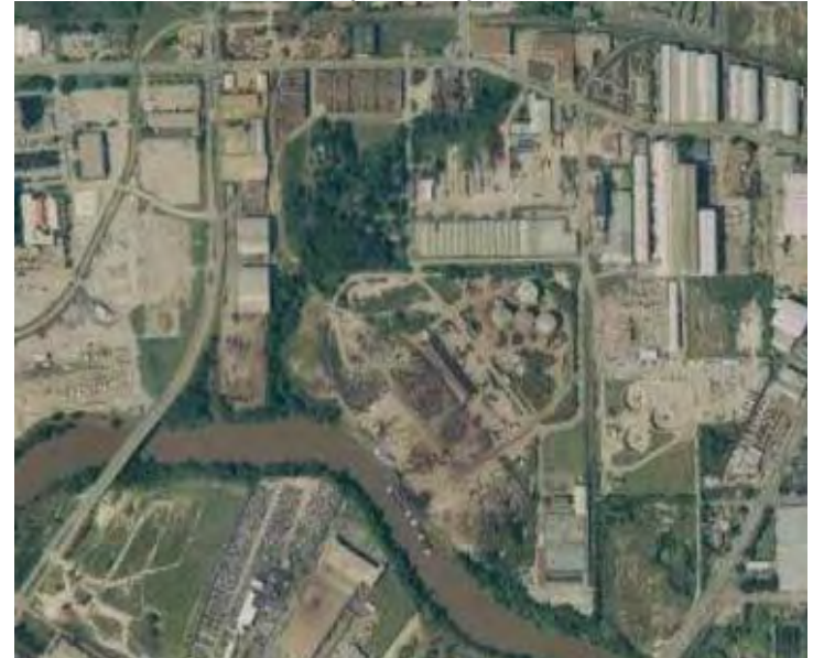
Aerial view of Zone 3 in the Buffalo Bayou Study Area
