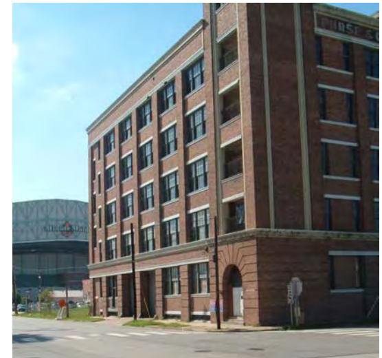
Silvestri condominium project
