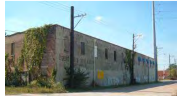
Basic Wire & Cable building
